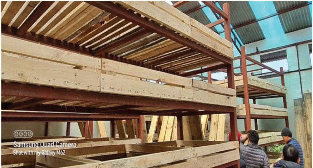
Fig.3: Showing horizontal plank gap, vertical tray gap for air circulation & fiber glass for diffused light system
